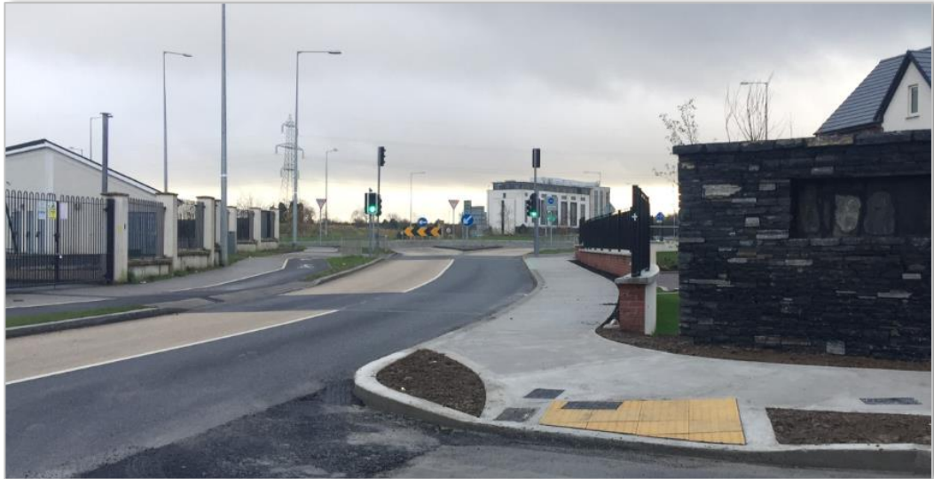
Figure 2.14: Existing Toucan Crossing on the R121
