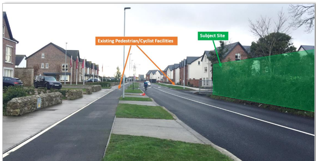
Figure 2.13: Existing Pedestrian & Cyclist Facilities on the R121
