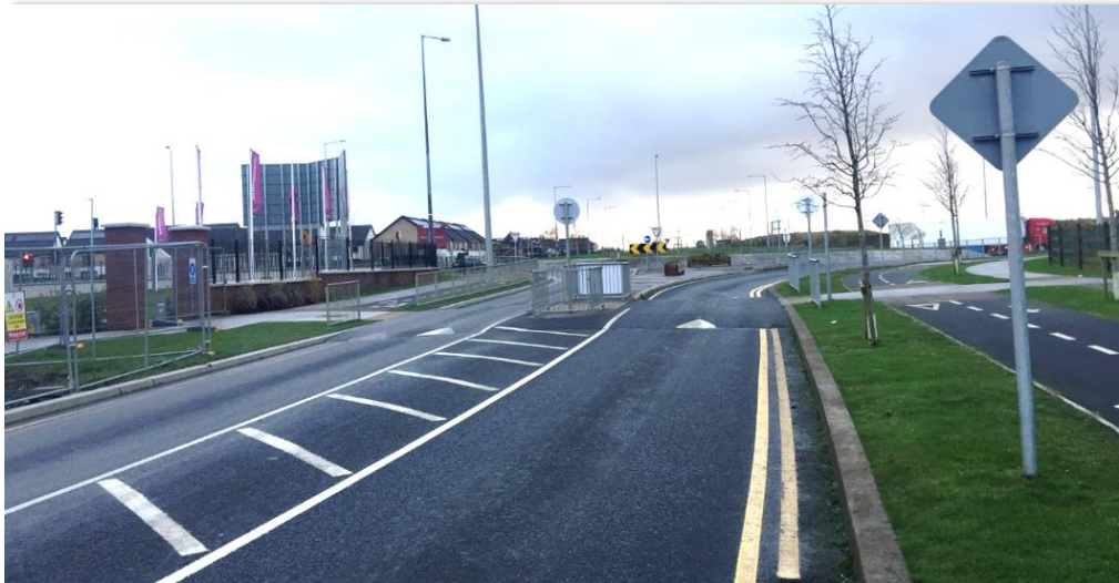
Figure 2.6: View Looking East on The Avenue Towards R121 Roundabout
