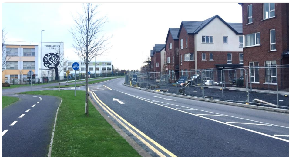
Figure 2.5: View Looking West on The Avenue Towards the Subject Site
