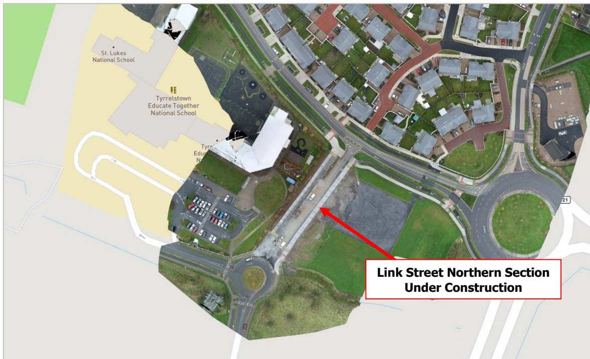
Figure 2.22: Aerial Image of Link Street Northern Section Under Construction (Image Taken 30 November 2021)
